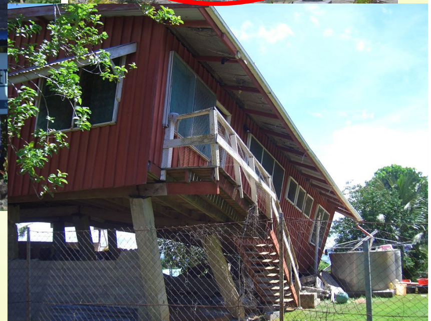
Damaged house on a hill in Gizo
